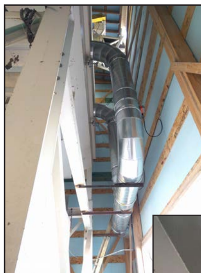
Heating Ducts Going into Aggregate Bins
