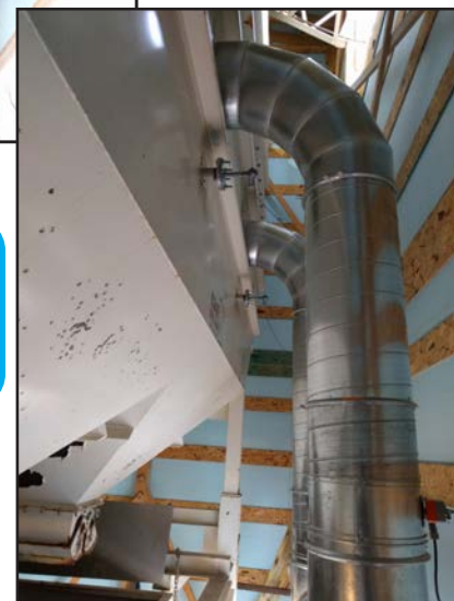
Heating Ducts Going into Aggregate Bins
