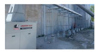
Sioux's Aggre-Flo® aggregate heater is designed to heat coarse and fine aggregates to eliminate ice and frozen chunks during winter. The entire aggregate bin is heated to a consistent temperature with dry heat that does not introduce moisture into the aggregate. This allows ready mix producers to keep aggregates flowing from their bins and get consistent batch quality, even during the coldest months.
